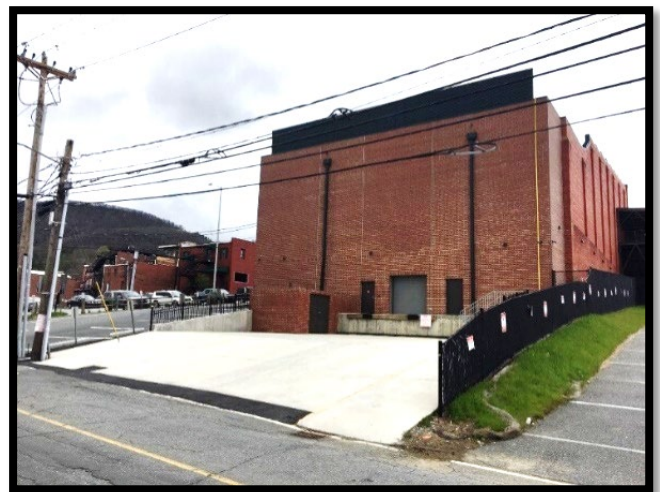
Loading dock facing North from Howard St
